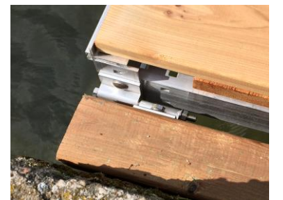
Ramp to Shore Hinge
